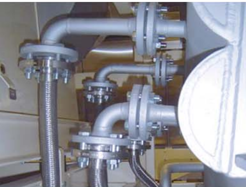
Flexible Steam and Condensate Interface
