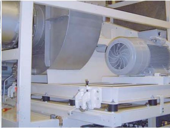
Fan and Heat Exchanger are installed on pull-out rails for maintenance.
